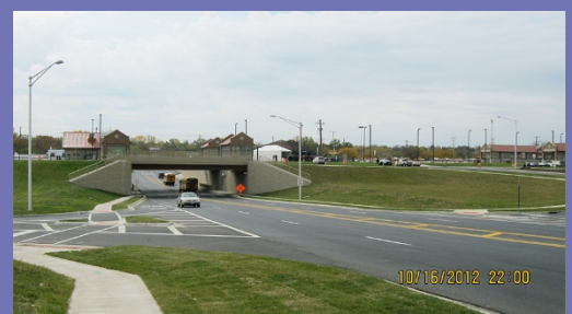
A recently completed CREATE grade separation in Downers Grove on Belmont Road at the BNSF Railway
